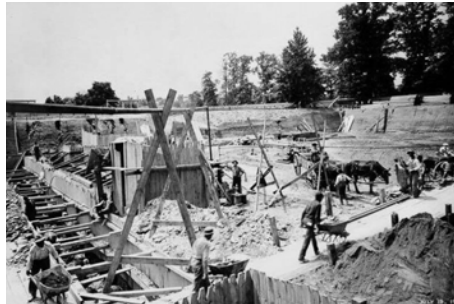
Below: CMA Masonry Begins
