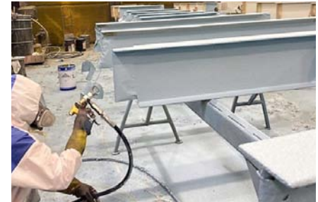
Above & Below: S-W Fireproofing Spraying on Steel Beams Bottom: Champion Infrastructure's Web Page on S-W HQ Fireproofing Contract
