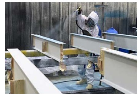
Above & Below: S-W Fireproofing Spraying on Steel Beams Bottom: Champion Infrastructure's Web Page on S-W HQ Fireproofing Contract
