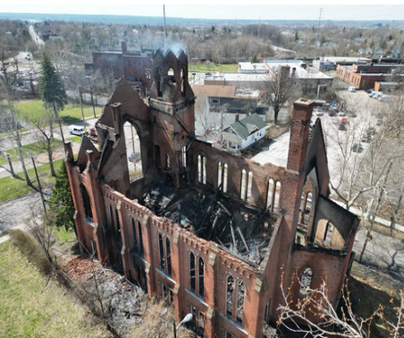
Below: Miles Pentecostal Determine Church after Fire
