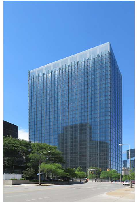
Above: Celebrezze Federal Building after the Facade Addition; Interactive Design; Chicago Below: Celebrezze's original design and construction; Shafer Flynn & Van Dijk with Dalton Dalton Little & Newport and Outcalt Guenther Rode & Bonebrake; 1969
