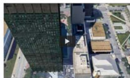
Erieview Tower and Galleria
