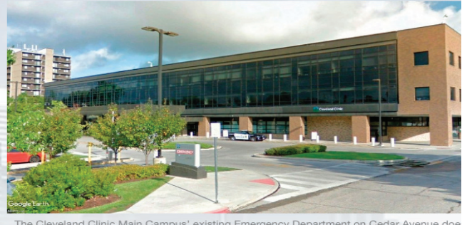
The Cleveland Clinic Main Campus' existing Emergency Department on Cedar Avenue does
