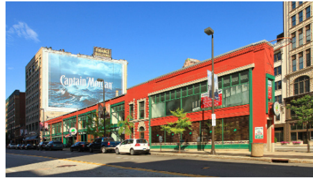
Above: Vacant 811 Huron Road
